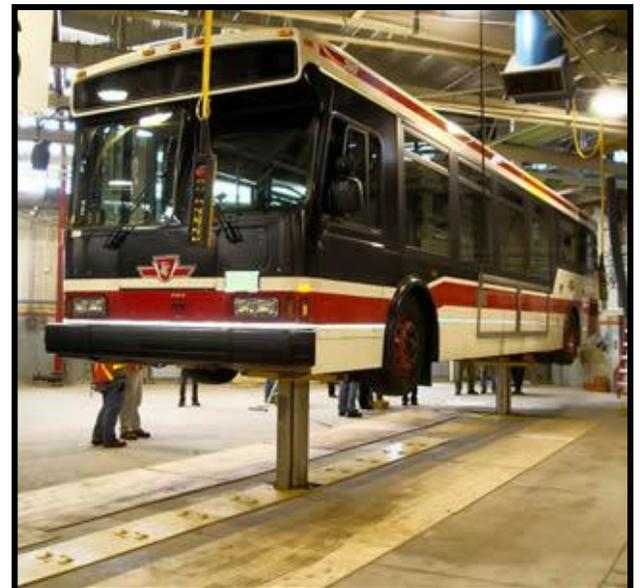
Latest high pressure installation of a bus hoist at **Toronto Transit Commission** facilities.
